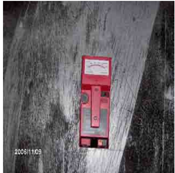
Roof 5 The roof was also checked with a capacitance moisture meter.
