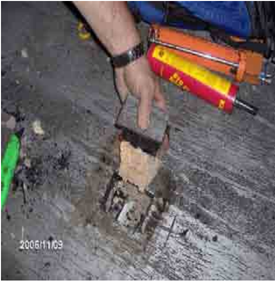
Roof 5 Core sample was dry.
