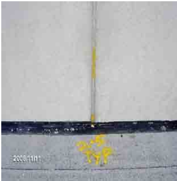
Roof 2-5 Apply sealant to joints.
