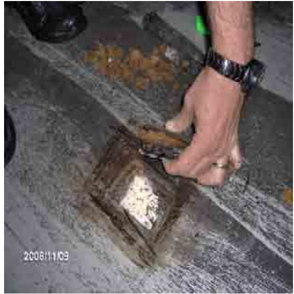
Roof 4 Core cut.
