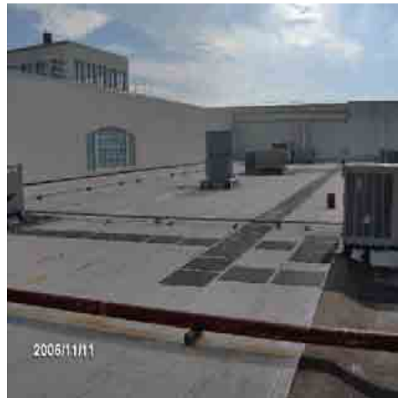
Roof Section 2 Overview of this roof section. Roof 1 is the high roof to the left.
