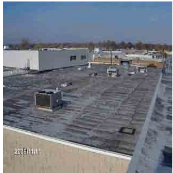
Roof Section 5 Overview of Roof 5.
