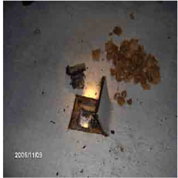
Roof 3 Core sample.
