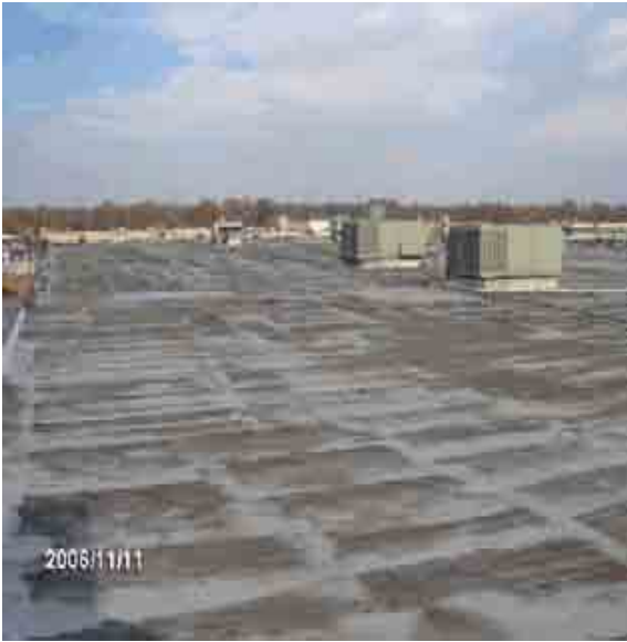
Roof Section 4 An overview of this roof section.
