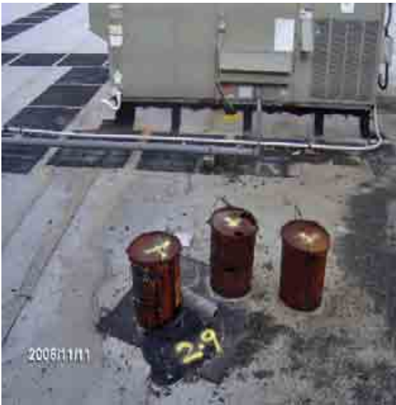
Roof 2-9 Remove all debris from the roof.
