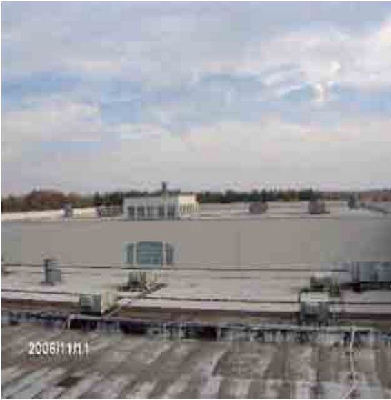
Roof Section 1 The high roof is in the distance.
