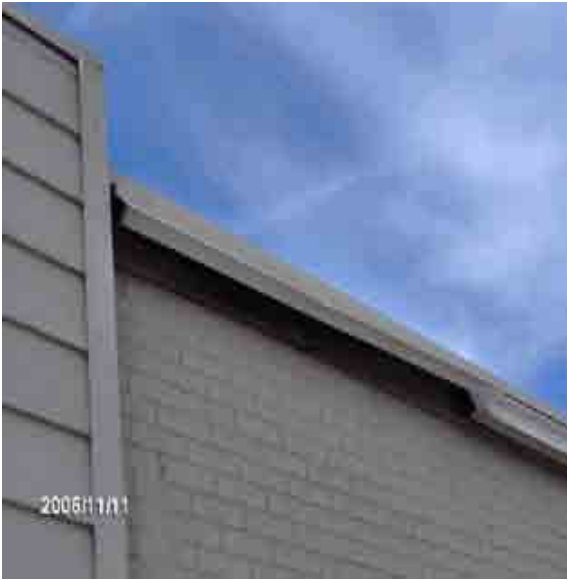
Roof 4-4a This is the metal as seen from below.
