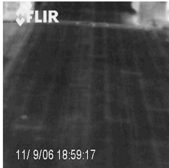
Roof 2-12 Another infra-red overview of Roof 2.
