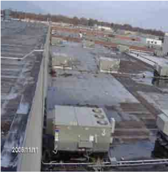
Roof Section 3 Overview of roof section.
